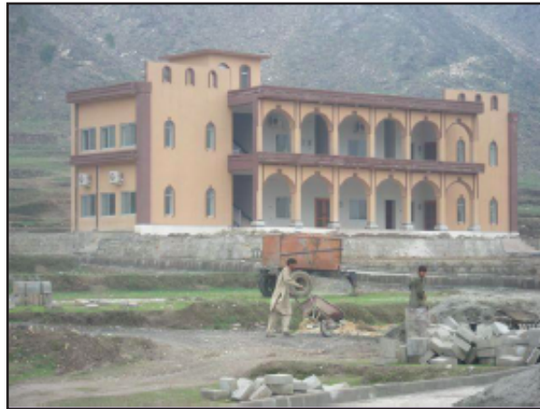
(Work going on around the herbarium)
